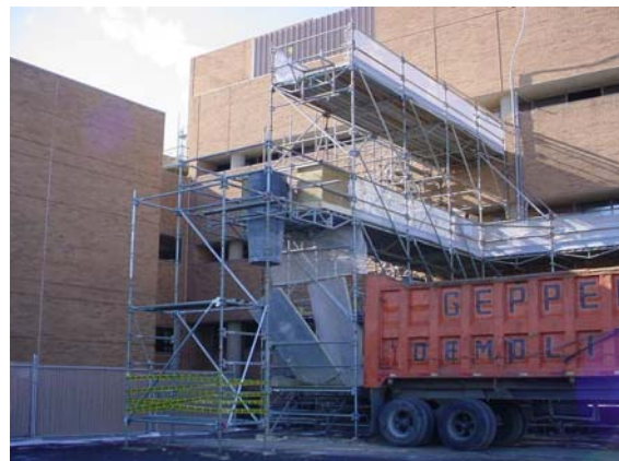
Recycling tubes outside AstraZeneca's lab renovation project in Wilmington.
