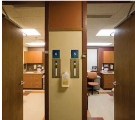
This side-by-side comparison of identical rooms shows the difference in lighting between the energy efficient bulbs (right) and original lighting (left) after retrofitting light fixtures in six buildings. The more efficient fixtures produce the same intensity light with more natural color and half the energy.
